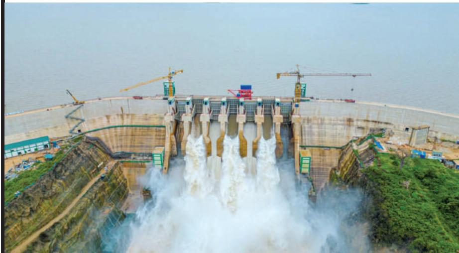
The final turbine was activated in April on the Julius Nyerere Hydropower Plant in Tanzania. Built by the Arab Contractors (**No. 93**) in JV with Elsewedy Electric, the project required 2.6 million cu m of concrete with 4 million cu m of excavation. The plant has installed power capacity of 2.1 GW. Tanzania had only 1.6 GW as of 2021, says the U.S. International Trade Administration. ■
