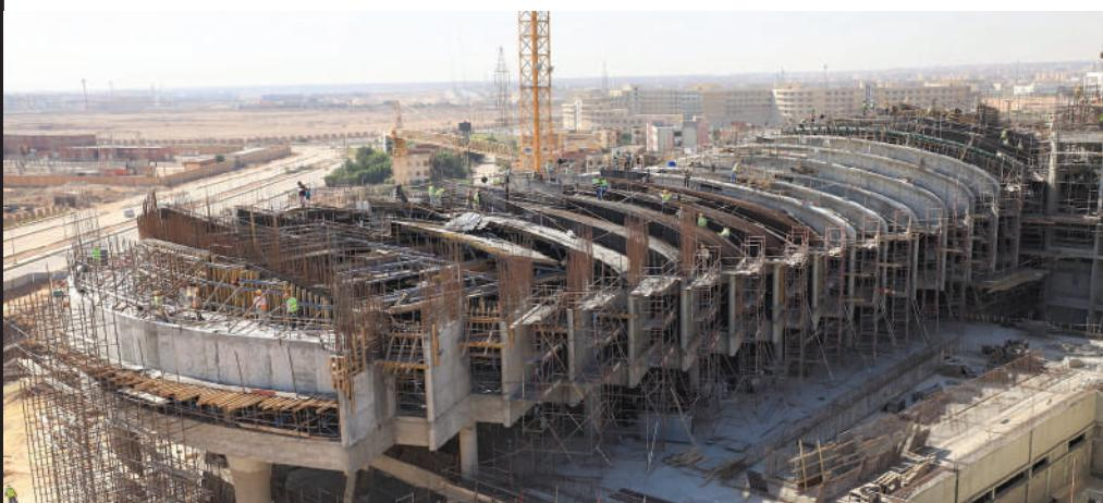
Orascom Construction (No. 40) is finishing work on the Magdi Yacoub Global Heart Center in Cairo. Designed by Foster + Partners, with EHAf and DAR consulting, the hospital will feature 88 concrete curved sections spread across four roof segments. The team used a 12-axis robotic formwork system to create the sections. The 85,000-sq-m facility is expected to host 120,000 patients annually, free of charge. ■
